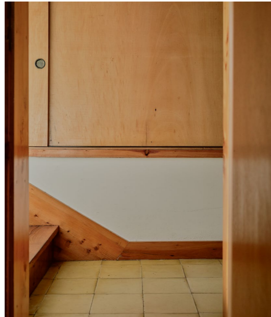
Wooden walls help to naturally regulate the temperature of the house. Wood has low thermal conductivity, meaning it both gains and loses heat slowly.
